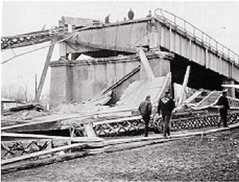
Figure 1.12: Section of U.S. 35 Silver Bridge that collapsed in 1967 due to crack propagation associated with residual stresses (photo courtesy of U.S. Dept. of Transportation, Federal Highway Administration).
